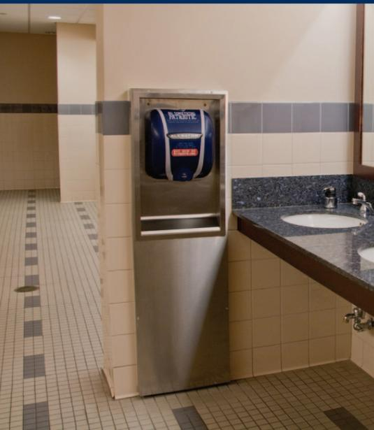
To further simplify the retrofit process, Excel Dryer provided the operations team with recessed wall boxes that allowed the dryers to be mounted precisely into the space where the paper towel dispensers once were.
